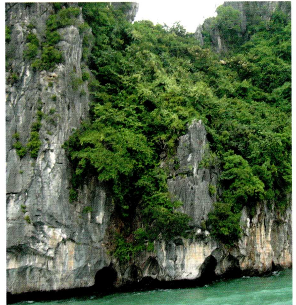
Photo 5: Foot caves and notches
